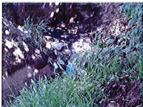
Garbage blocking a water tunnel
