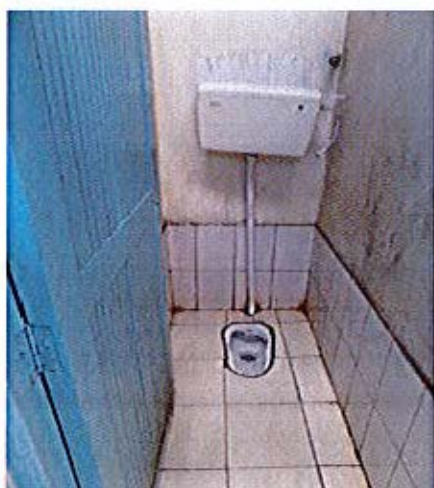
One of the public toilets constructed
