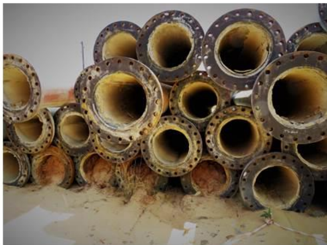
Pipes that carry the harmful water from the mines and tailings to dam sites are littered around the lands. As the photographs show they are layered with the sediments of the heavy metals.
