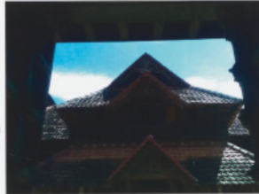
Poomukham roof seen framed by the Padippura
