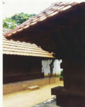
The curved brackets of roof overhang
